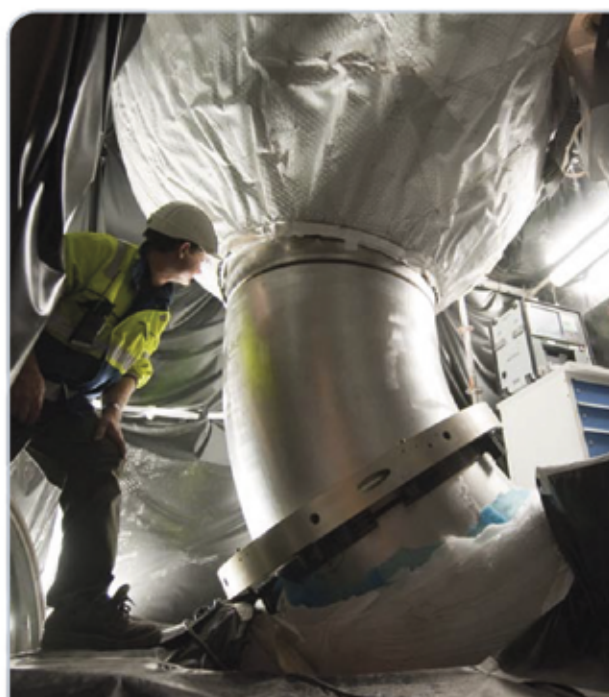
Aligning of a cross-over leg.
