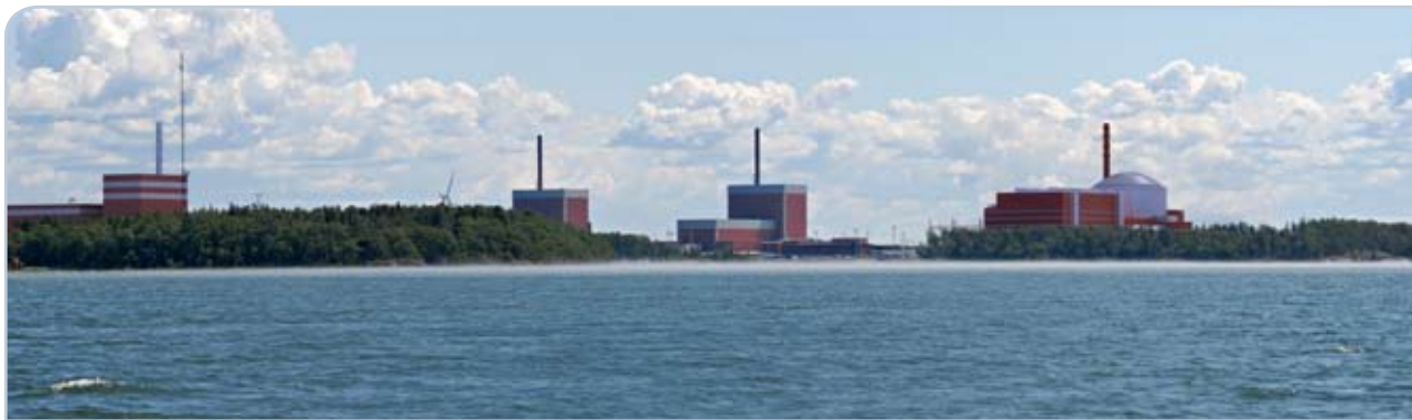
Figure 9-29 Olkiluoto island seen from the sea. The photomontage shows the existing plant units OL1 and OL2, the OL3 plant unit currently under construction in its completed form and OL4 on the left.
