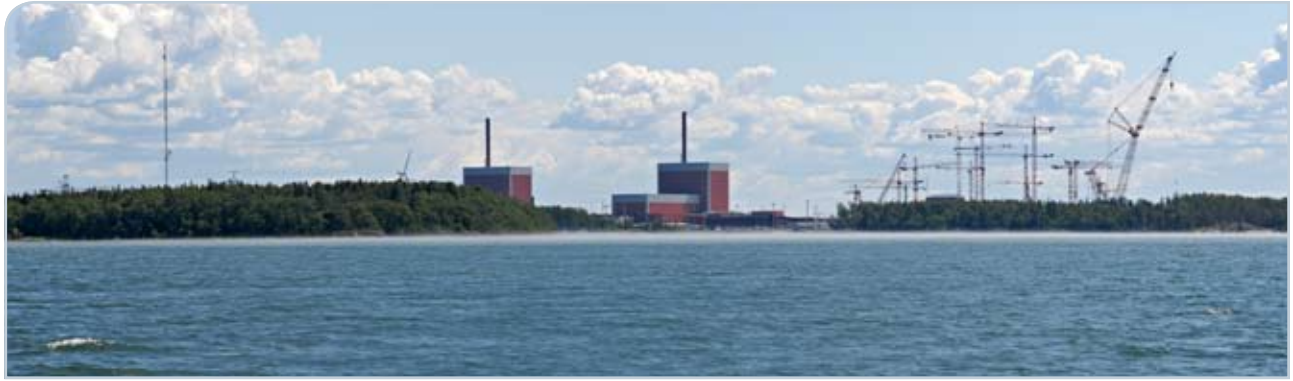
Figure 9-28 Olkiluoto island seen from the sea. The existing plant units OL1 and OL2 and the OL3 construction site on the right.
