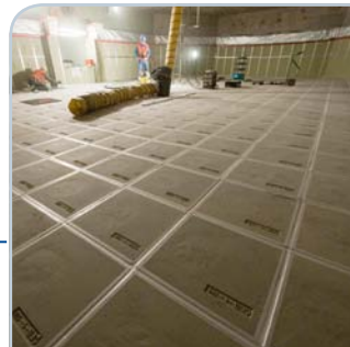
Core melt spreading area
