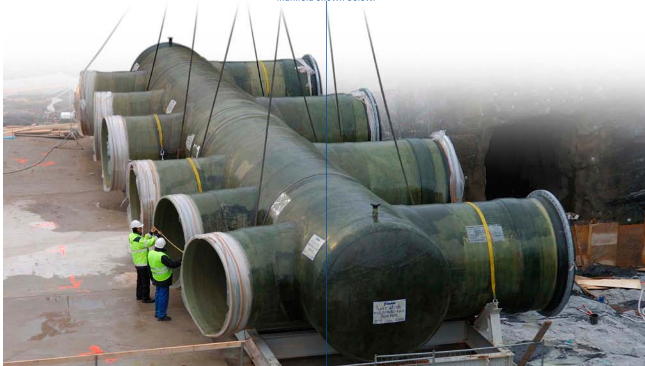
The cooling water pumped by the sea water pumps is conveyed into a sea water condenser through the manifold shown below.
