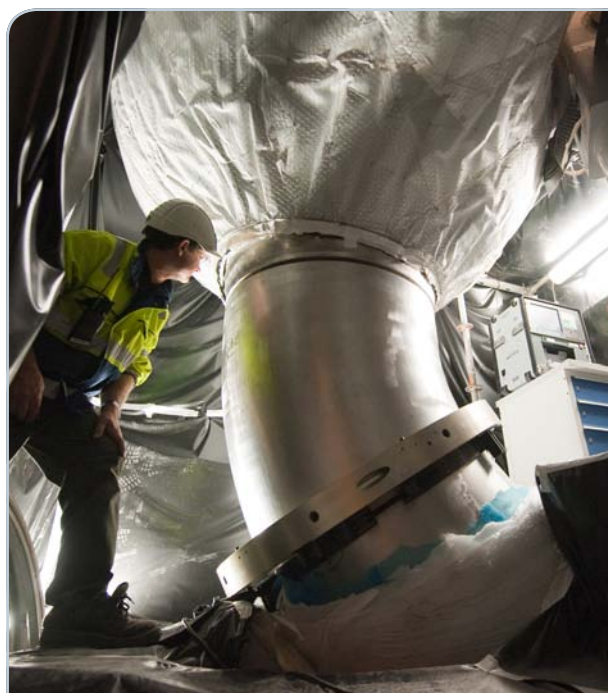
Aligning of a cross-over leg.
