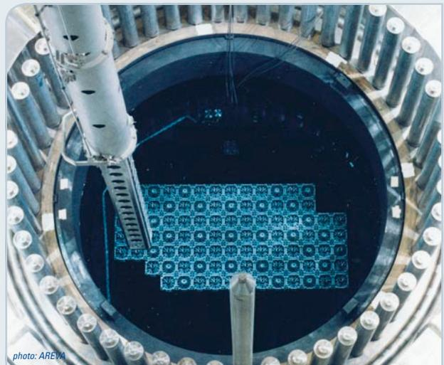
An essential matter in the reactor operation is the correct positioning of the fuel assemblies that vary in age and power. A uniform power distribution in the reactor guarantees a high safety level and a cost-effective fuel use.
