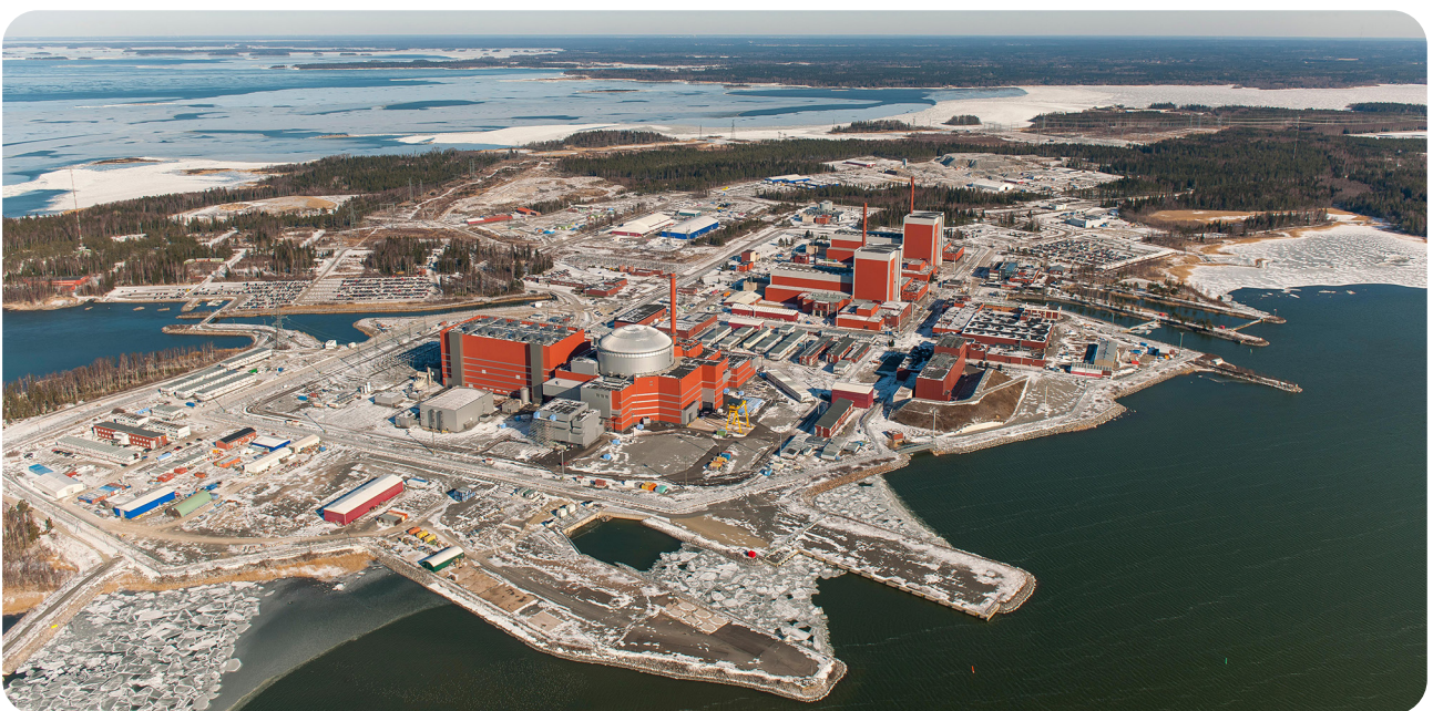
Figure 2. Aerial view of the power plant area.
