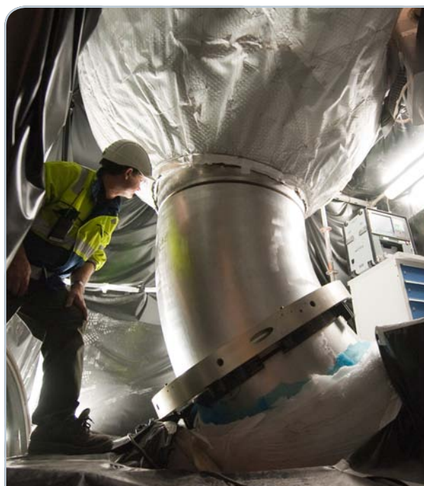
Aligning of a cross-over leg.
