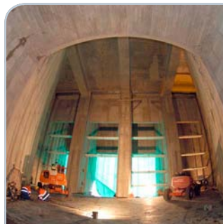
The cooling water intake tunnel has a cross-section of about 60 m 2 .
