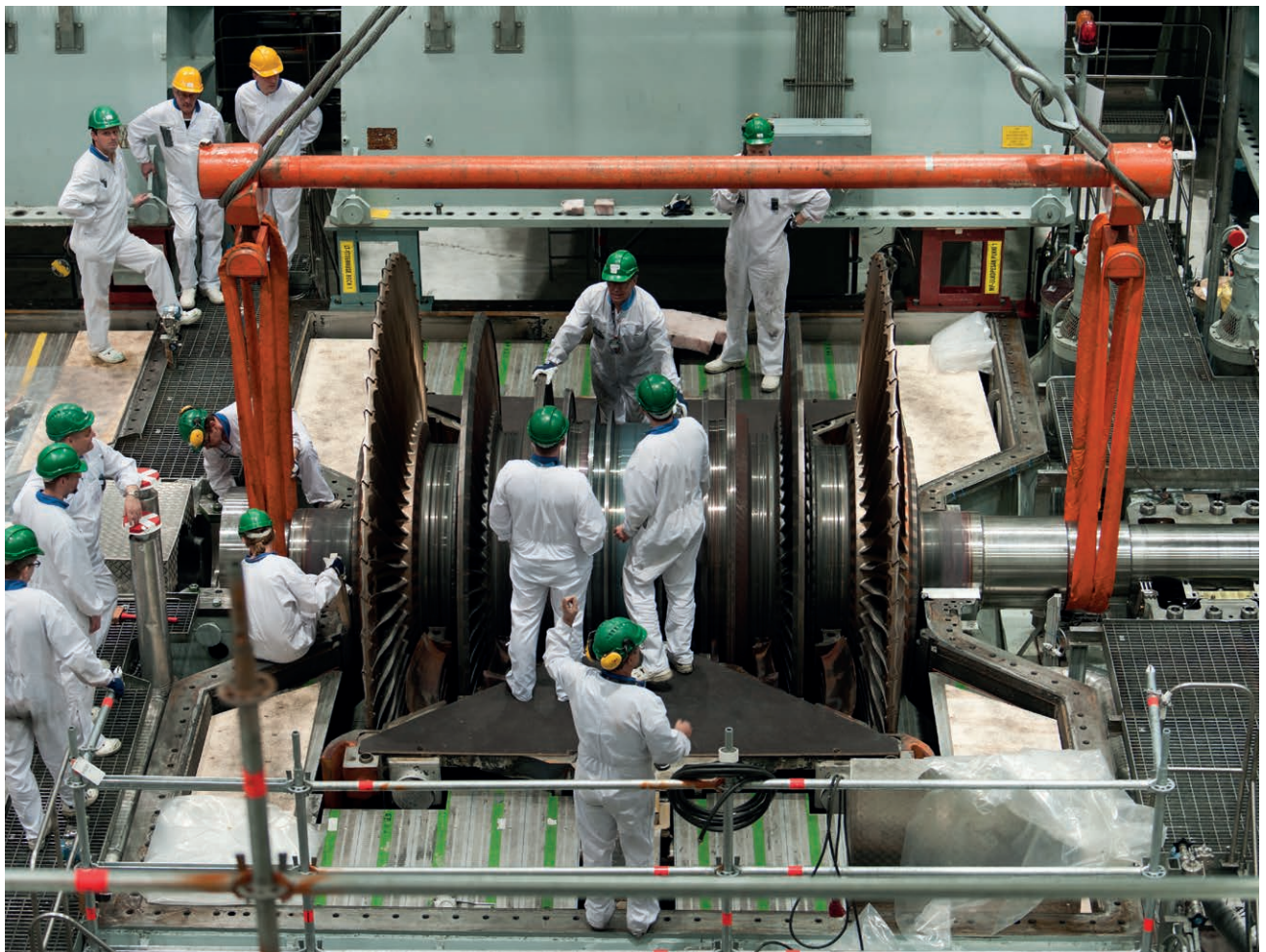
Low pressure turbine work inside the turbine hall.
