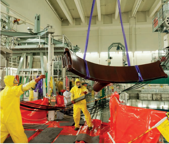
Moving a feedwater distributor for inspection requires special attention.
