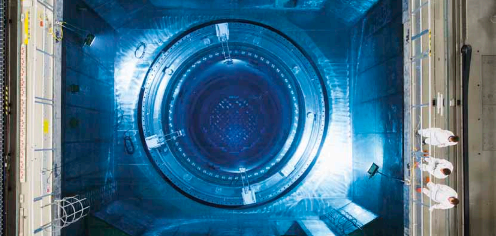
The reactor pressure vessel seen from above. The closure cover bolt holes on the pressure vessel flange are sealed with plugs. The closure cover is surrounded by the containment seal, which in turn is surrounded by the containment cover attachment flange.
