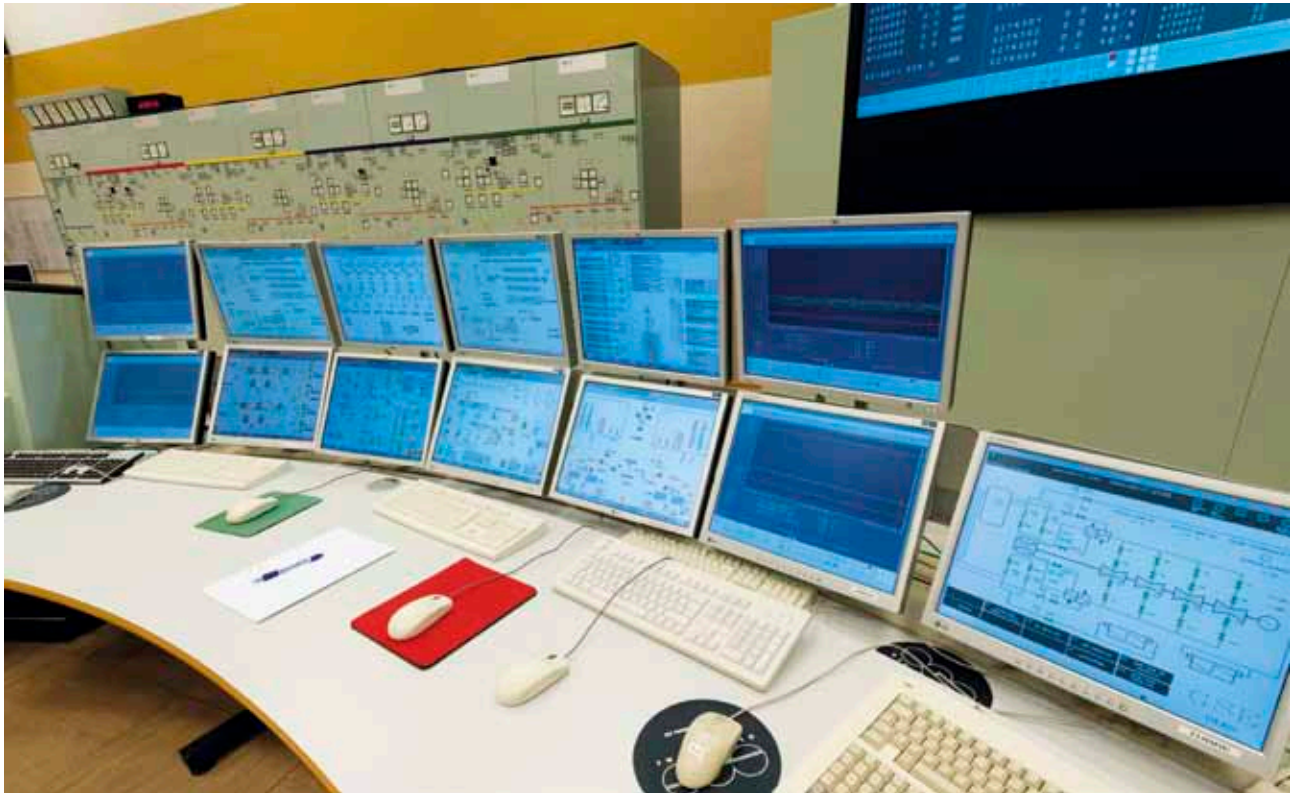
The turbine automation control and display workstations
