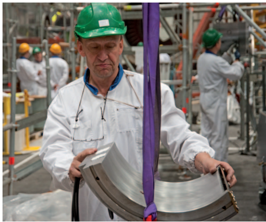
A turbine bearing segment has been inspected and cleaned thoroughly before being transferred into place.
