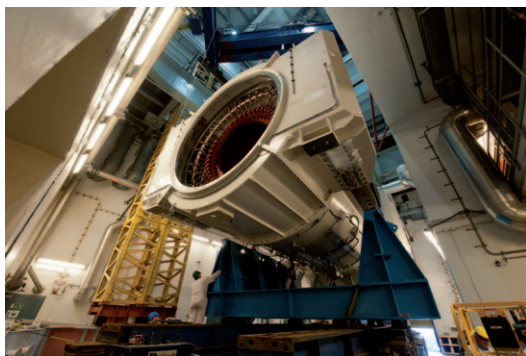
Lifting the new generator stator off the transport platform.
