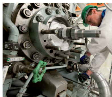
The annual service for the feedwater pump included, among other things, the replacement of the slip ring seal and a complete condition inspection.
