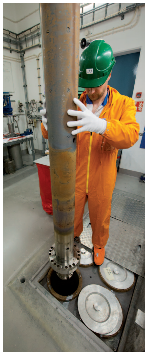
Jussi Juntunen, Sami Mäkinen, and Vesa Laakso from ALSTOM Finland servicing control rod drives in the service facilities.
