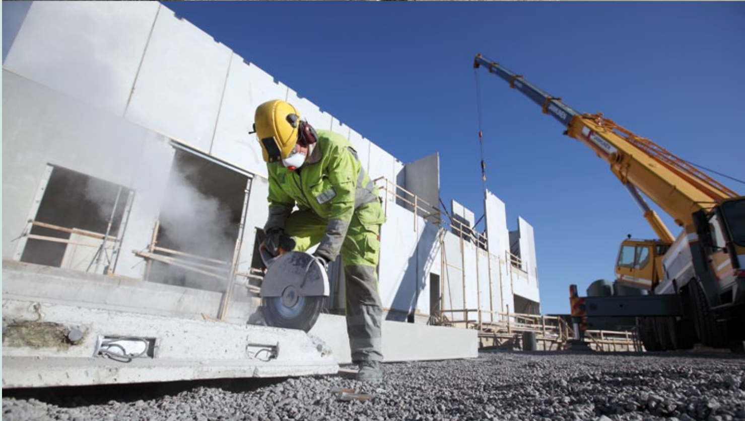
The ventilation building of ONKALO reached its full height in late 2010.
