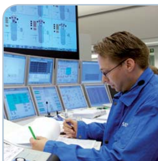
A shift supervisor and operators, all holding a licence for operating the plant, are present in the control rooms of the units at all times.
