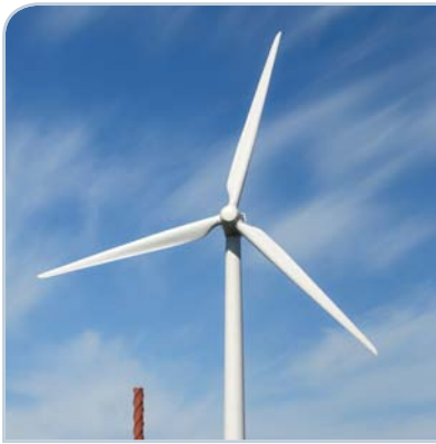
Olkiluoto's wind power plant generated 0.002 TWh of electricity.
