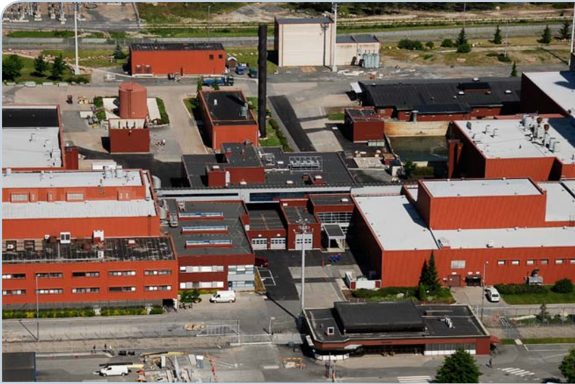
The annual outage building functions as a combined entrance for the power plant units. The building features a new radiation monitoring system based on double-monitors.
