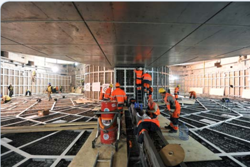
Work ongoing at the reactor containment; emergency cooling basin being constructed.
