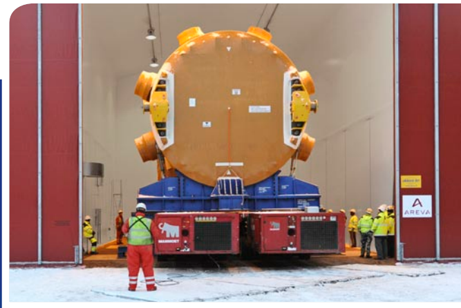
The reactor pressure vessel arrived by sea at Olkiluoto in early 2009.
