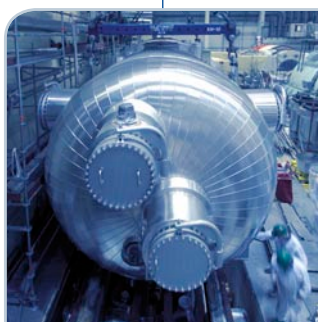
The OL1 reheater was changed in the annual outage.
